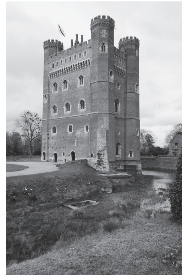
FIG. 2.21 Tattershall Castle, Lincolnshire, England, 1434–46.
