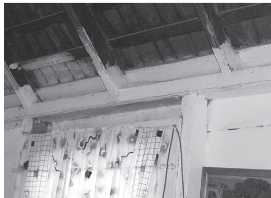
FIG. 8.3 Detail of wall plate, 54 Duke Street, Falmouth, Jamaica.
