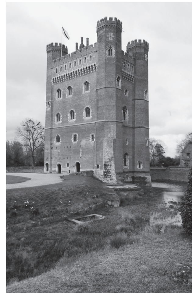
FIG. 2.21 Tattershall Castle, Lincolnshire, England, 1434–46.
